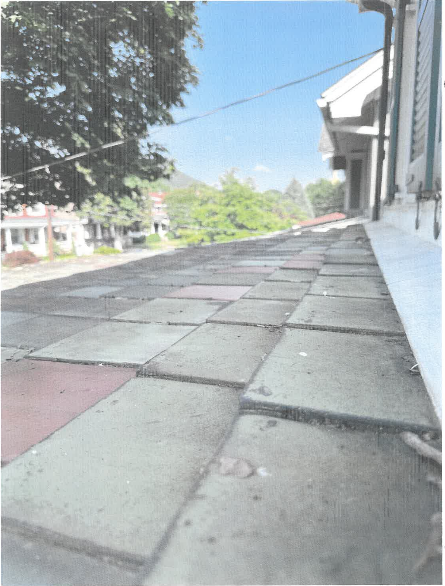
PORCH RIGHT SIDE
