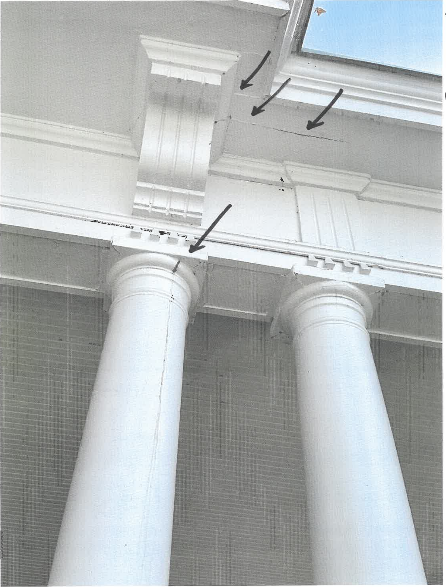
PORCH CENTRAL COLUMNS
