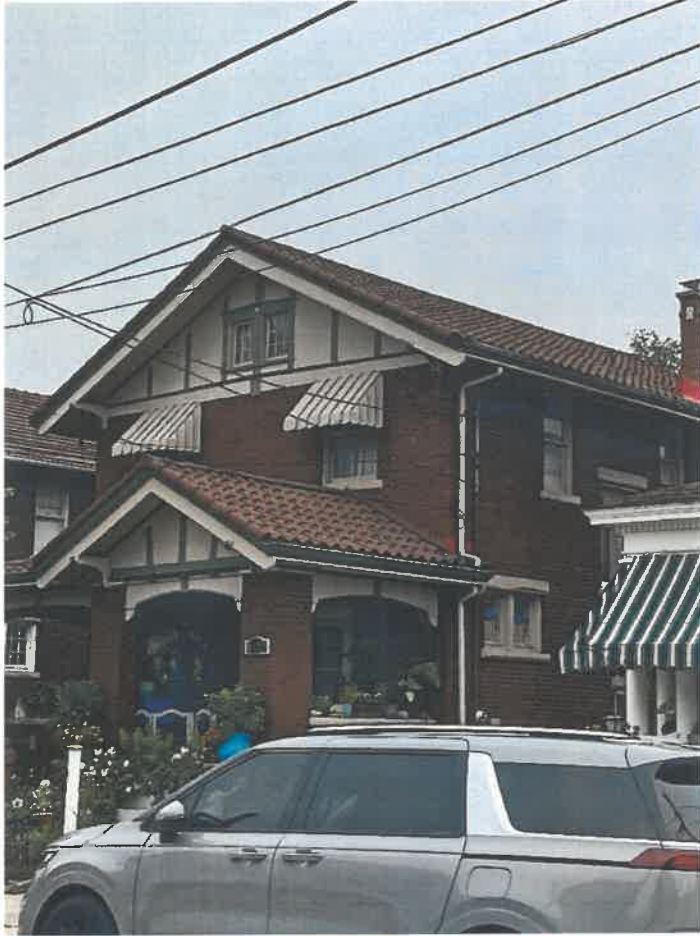
House at 1622 Quarrier St. E with similar tile that will be installed on our house.
