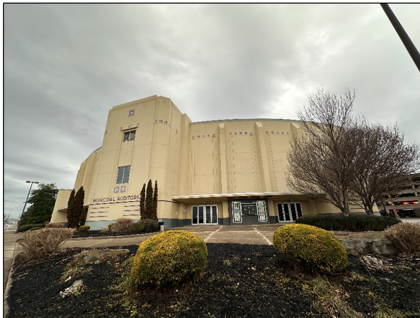
Photograph 1: Front Elevation – CIP Concrete Facade
