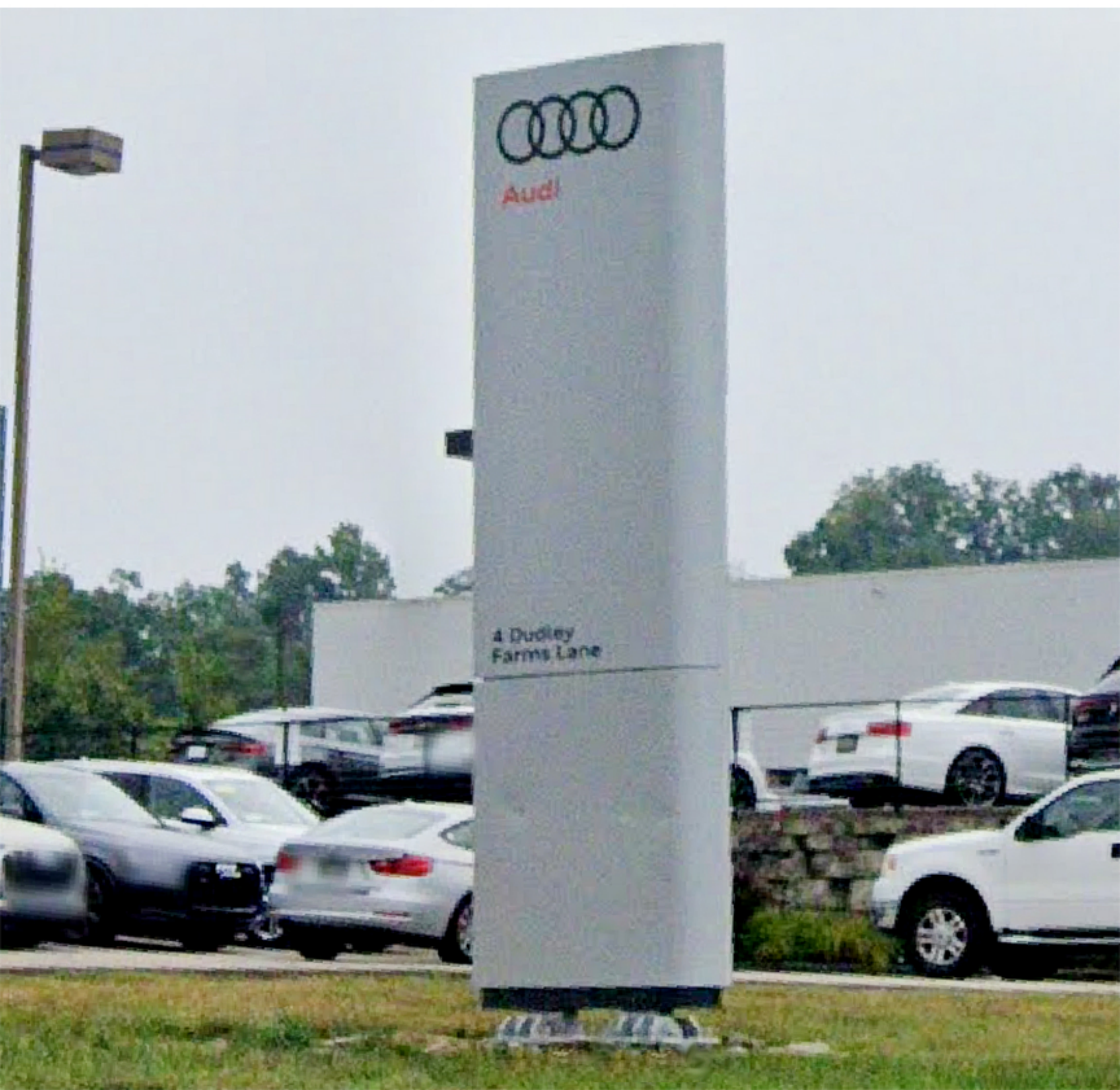
Audi Pylon Sign Close Up (needs to be replaced)
