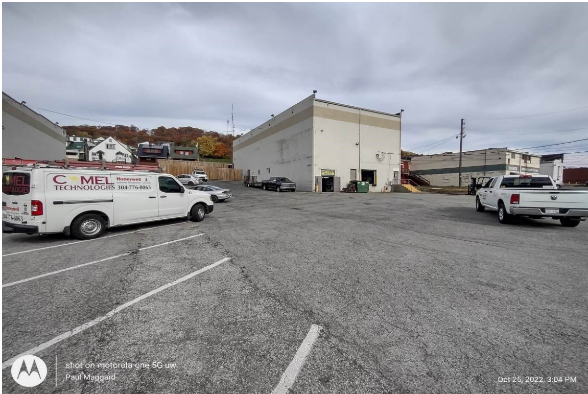
Photo 2: Looking NE Across Pile Off-Street Parking (October 25, 2022 at 1:00 PM)
