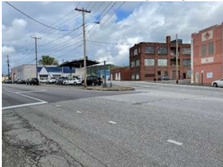
View, Central Avenue West Leg, Looking WB
