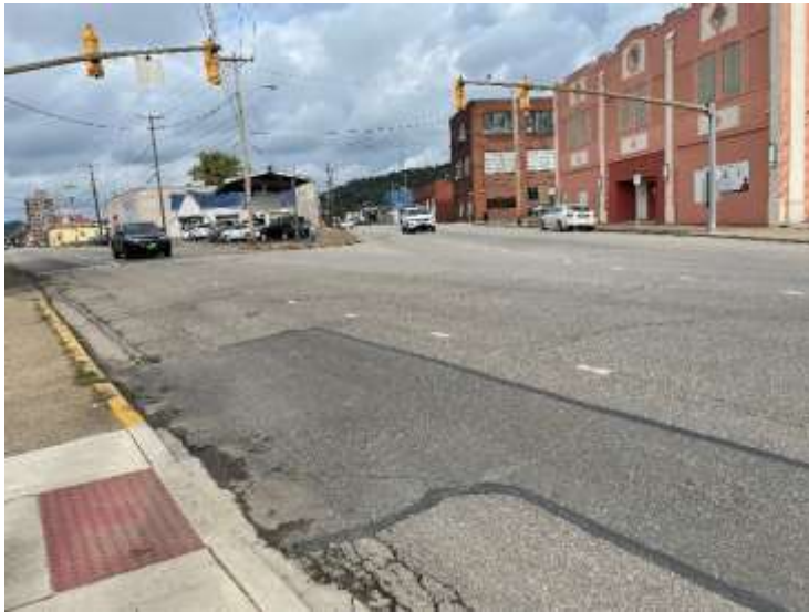
View, Central Avenue West Leg, Looking WB
