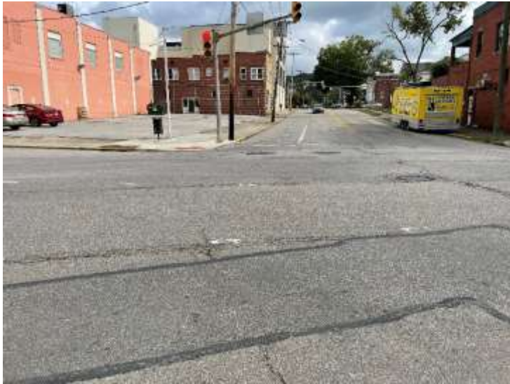
View, Delaware Avenue North Leg, Looking NB
