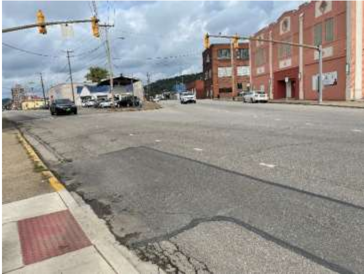
View, Central Avenue West Leg, Looking WB
