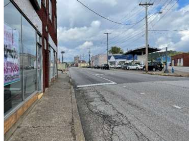
View, Central Avenue West Leg, Looking WB
