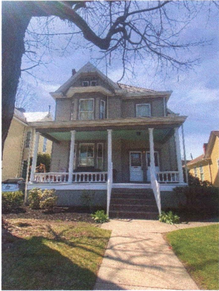
1411 Front view from Quarrier Street
