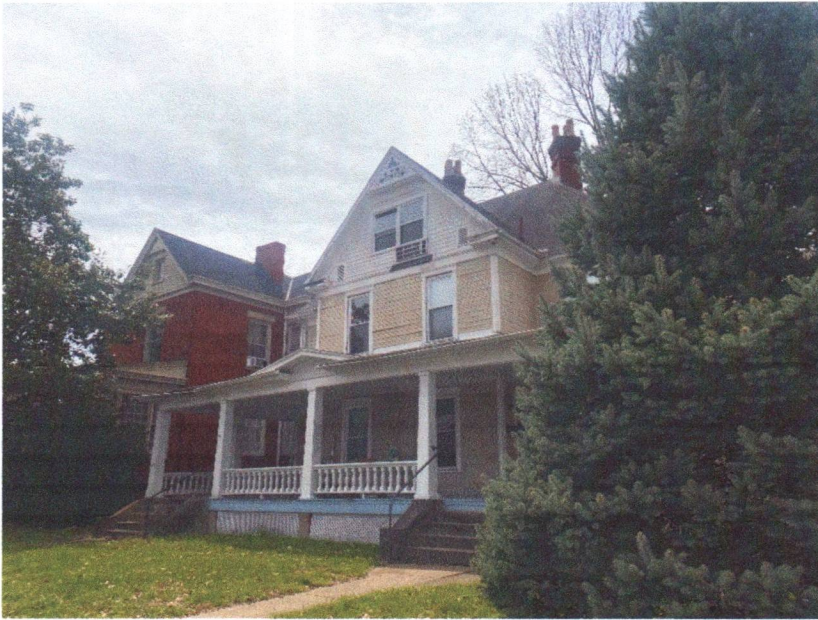
1415 Quarrier – Showing external guttering and standard shingles
