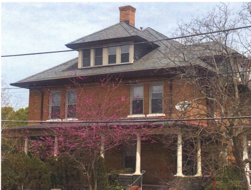
1410 Quarrier – Showing external guttering
