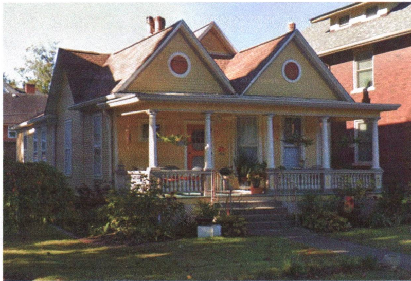
1409 Quarrier Street – showing external guttering and standard shingles
