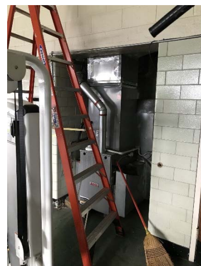
Split System Gas Furnace
