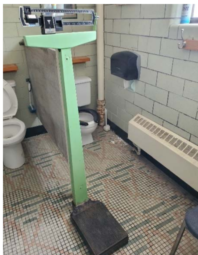
Existing Toilet Stall
