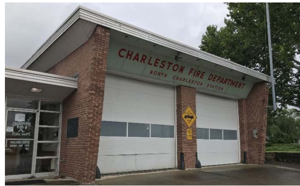
Former Vehicle Bay Doors
