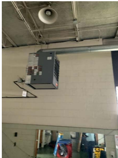
Suspended Gas Heater
