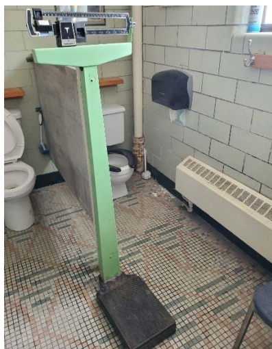
Existing Toilet Stall
