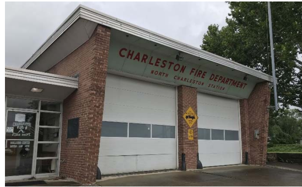
Former Vehicle Bay Doors
