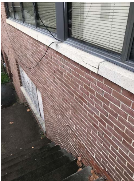
Damaged Windowsill
