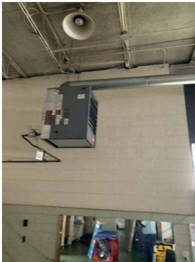
Suspended Gas Heater
