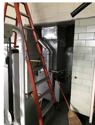
Split System Gas Furnace
