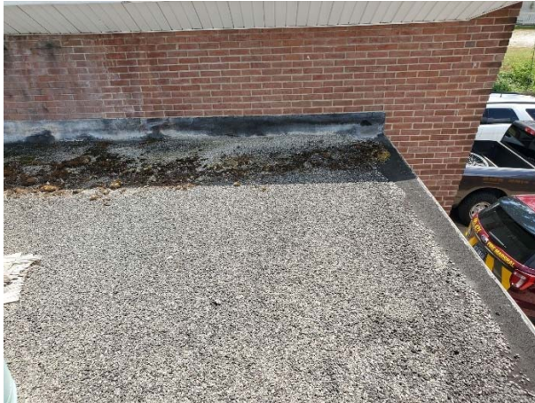
Existing Roofing and Flashing
