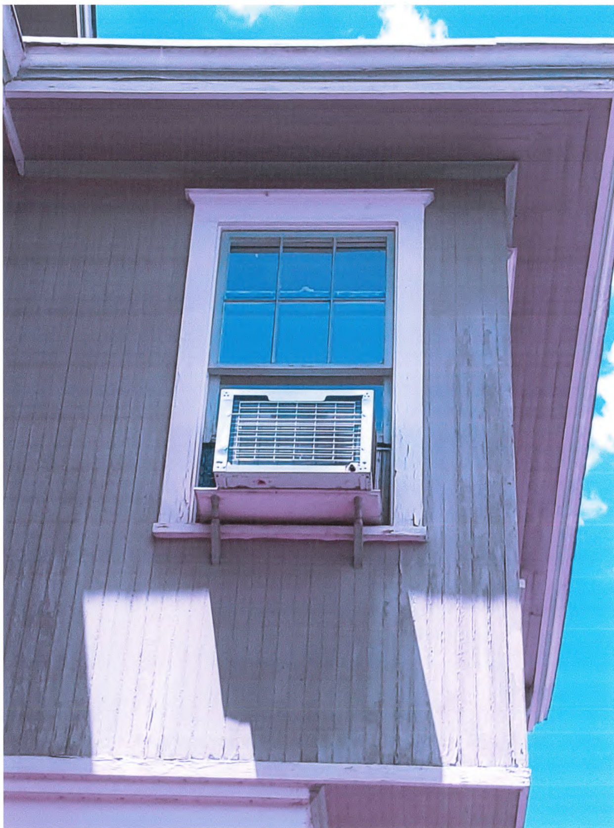
Exterior east facing sleeping porch window
