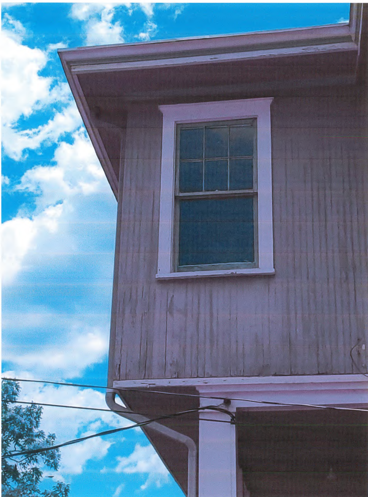
West facing sleeping porch window
