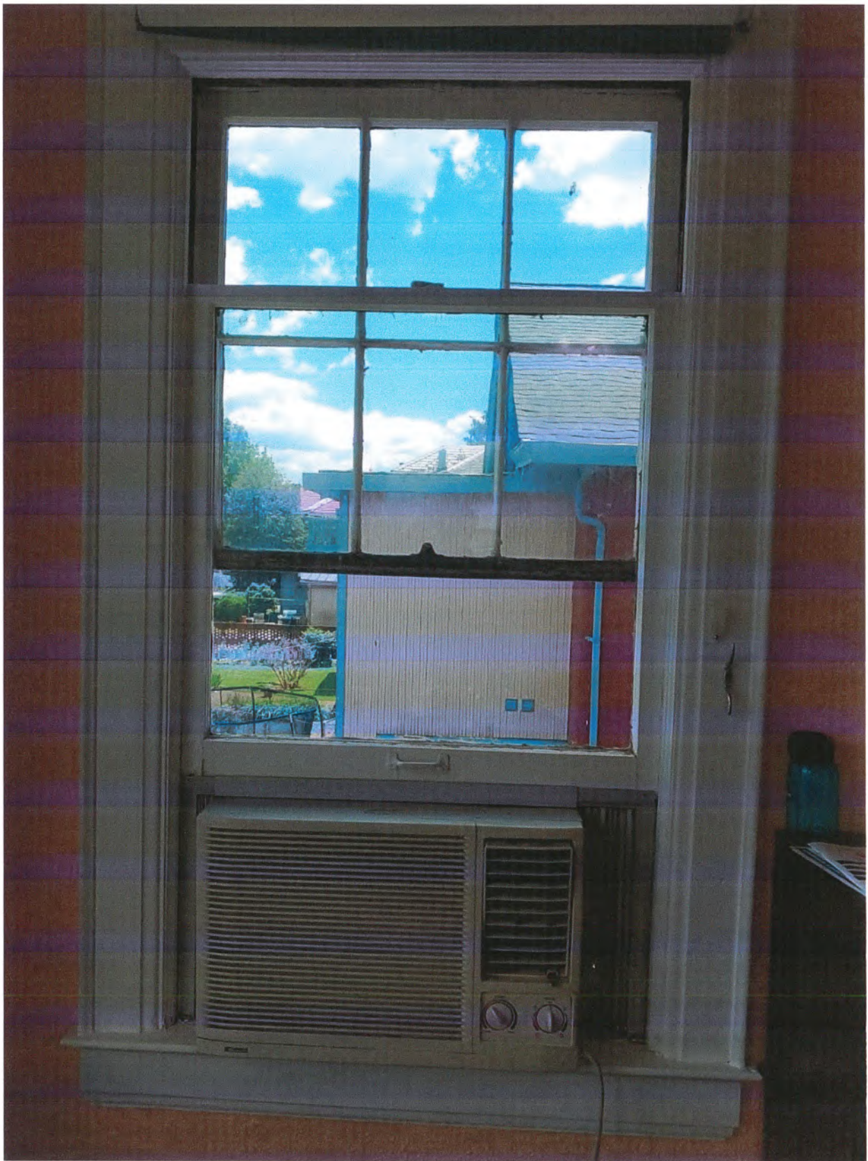
East facing sleeping porch window with combination A/C heating unit. With better insulation we are hoping to forego re-installing the A/C heating unit
